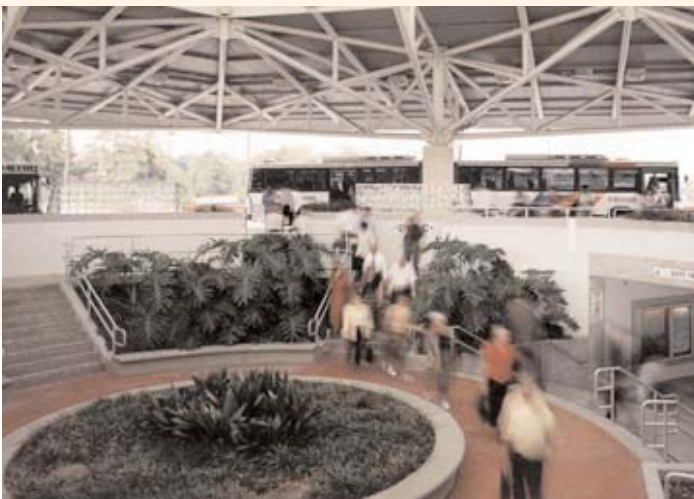
Many Metro riders catch their bus each workday from the Authority's 25 Park & Ride lots. These lots, including the Kuykendahl Park & Ride lot west of I-45 North, provide some protection from the elements and offer rides that run as often as every 5 minutes during rush hour.
